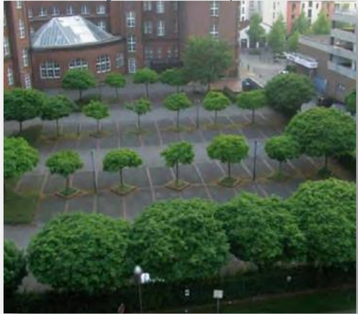
Figure 42 - Lack of soil volume and compaction has harmed the tree growth rates in this car park
